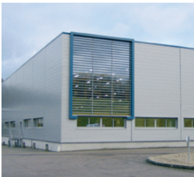
^ Controlled solar protection on an industrial building
